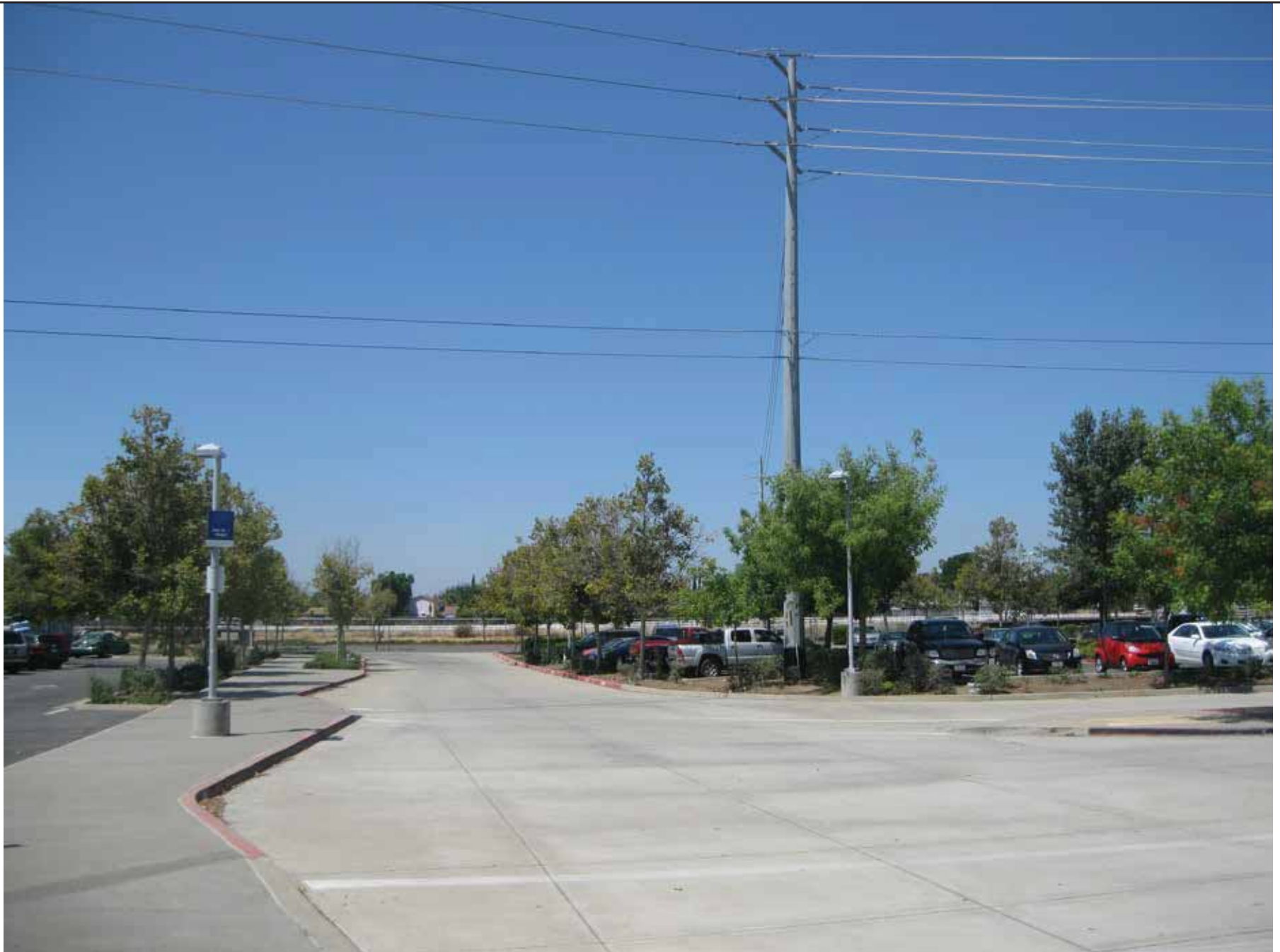
EXHIBIT 12: Point of beginning of proposed project, at the existing 69 kV TSP in the Meadowview LRT Station parking lot 69 kV Transmission Line and Joint Pole Facilities Relocation Project
