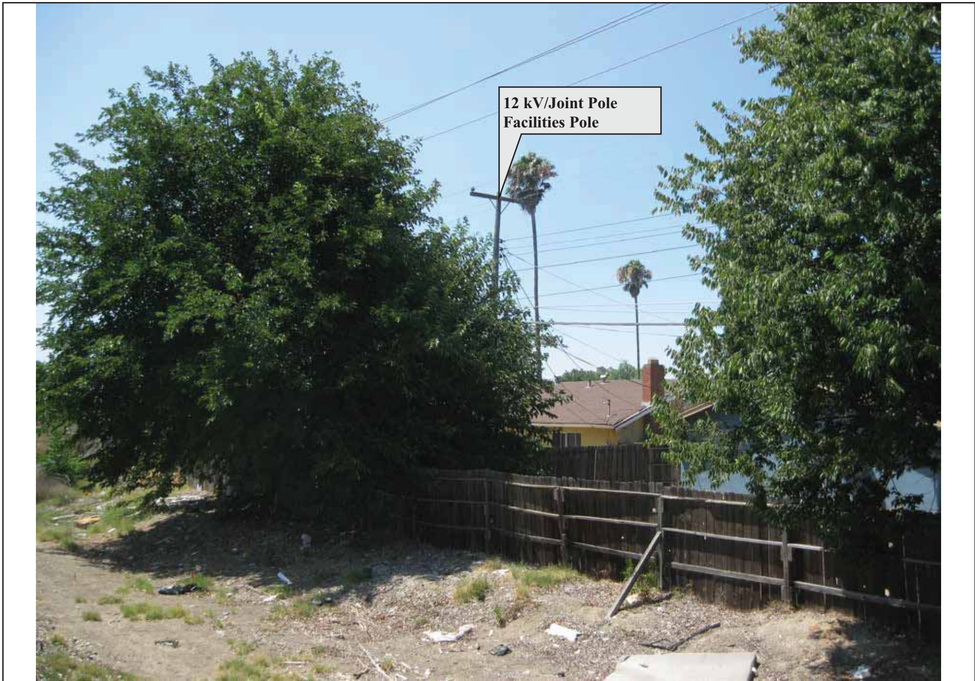
EXHIBIT 7: Typical existing backyard placement of a 12 kV/joint pole facilities pole
