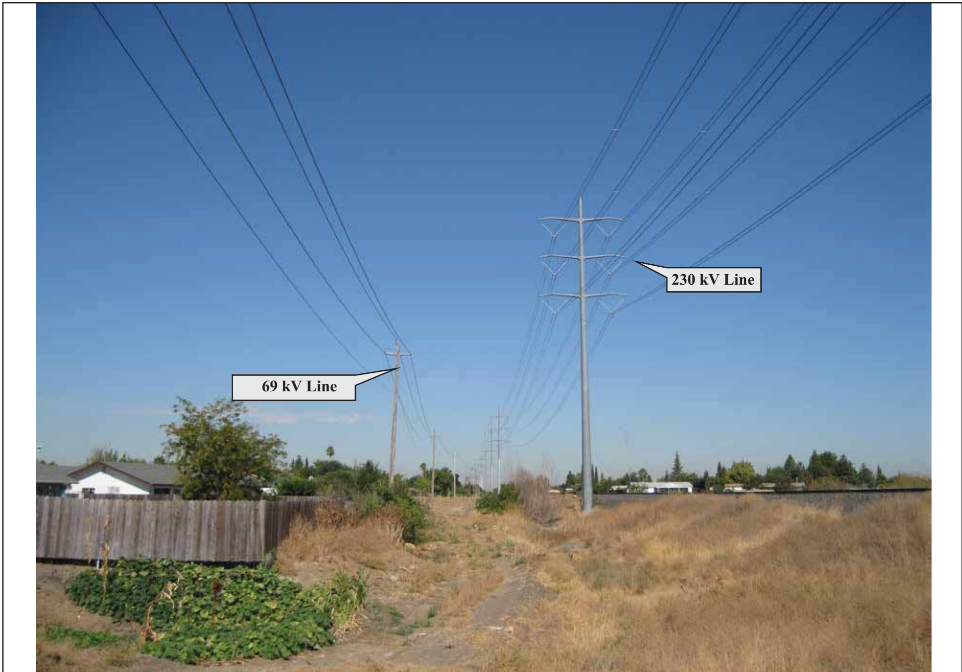
EXHIBIT 8: View looking north at future LRT alignment from vicinity of Morrison Creek
