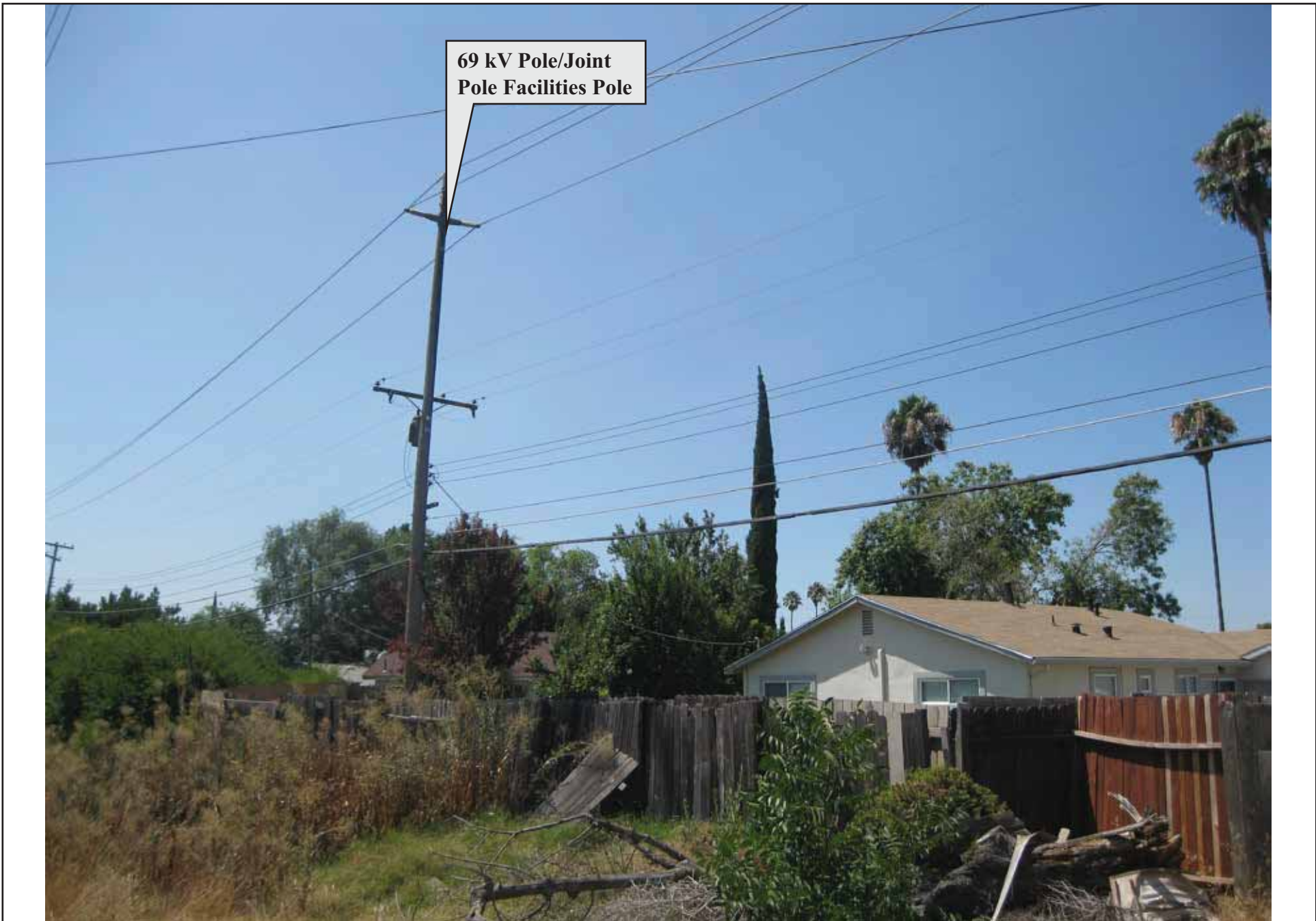
EXHIBIT 6: Typical existing backyard placement of a 69 kV/joint pole facilities pole
